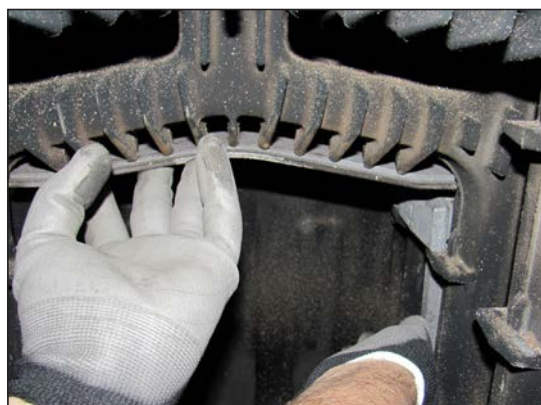
Fig. 5 2 nd deflector with the front side supports
